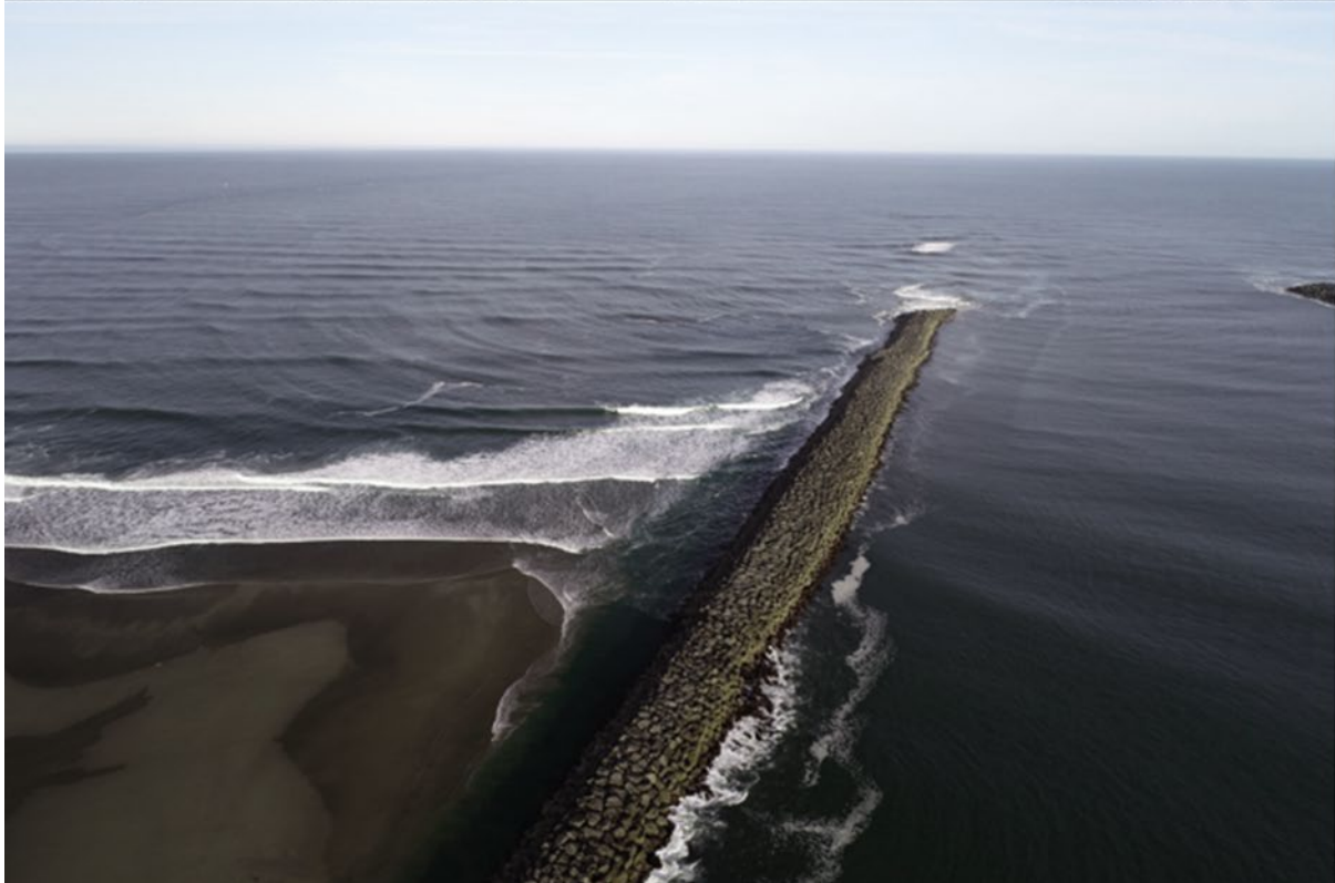
Figure 2. Existing Condition of the Tillamook South Jetty Head
