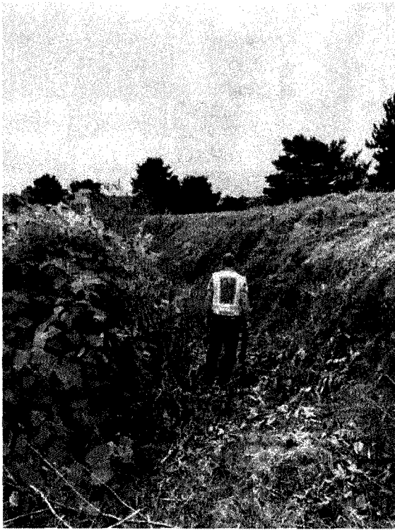
VERTICAL SLOPE STA. 8+25
