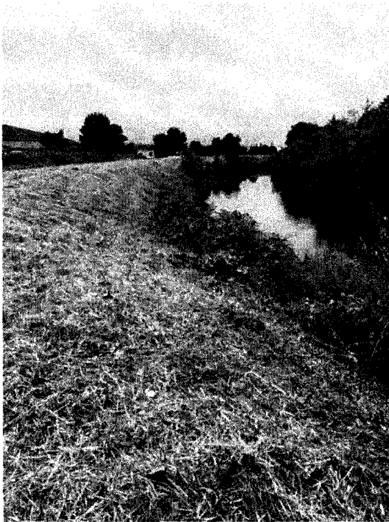
LOOKING DOWNSTREAM FROM STA. 1+50 APPROX.
