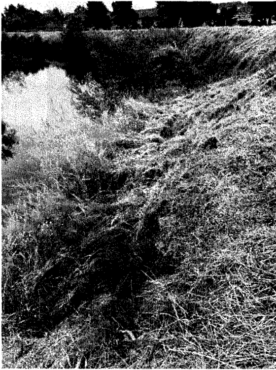
VERTICAL SLOPE BETWEEN STA. 7+00 AND 8+50 APPROX.
