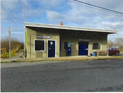
Oceanside Community Club roof repair $55,000
