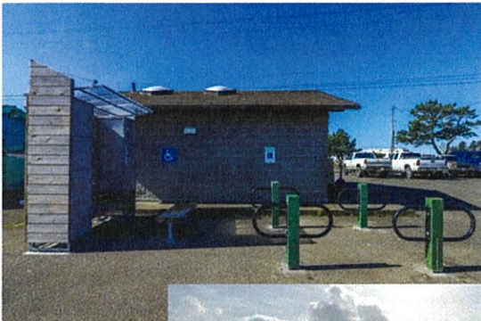
Restrooms and kiosk
