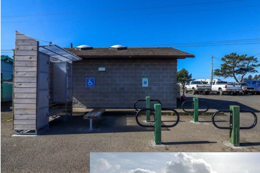
Restrooms and kiosk
