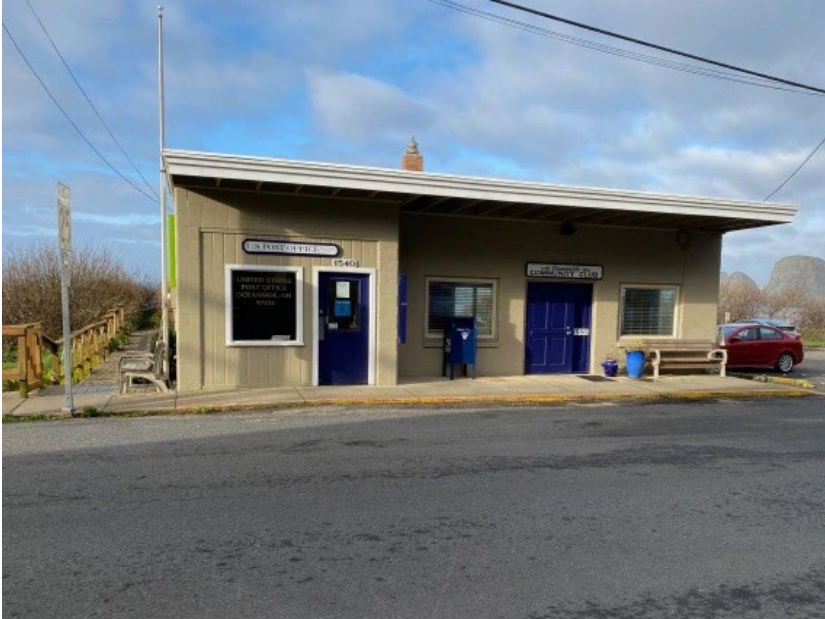
Oceanside Community Club roof repair $55,000
