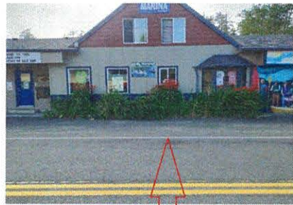
Building to the South (Kayak Shop) Sits 1.3' from the property line
