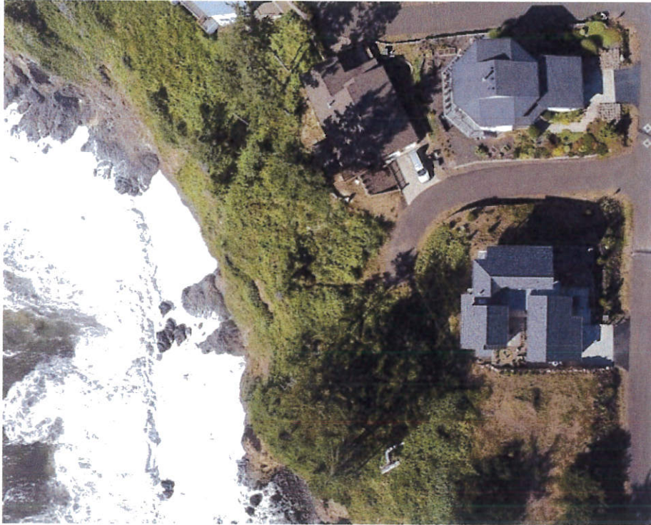
Photo 3 - Oblique aerial photograph of the site, nearby lots and the Pacific Ocean to the west.
