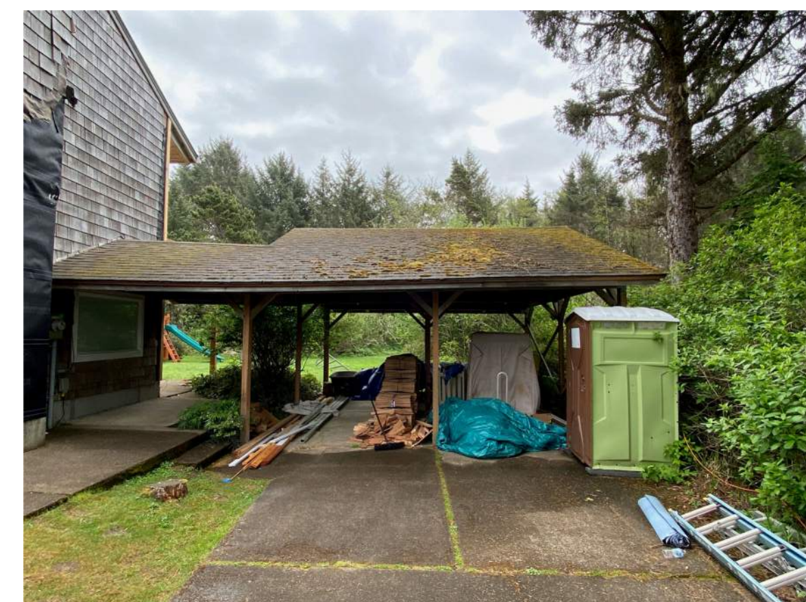
7 EXISTING CARPORT - FRONT
