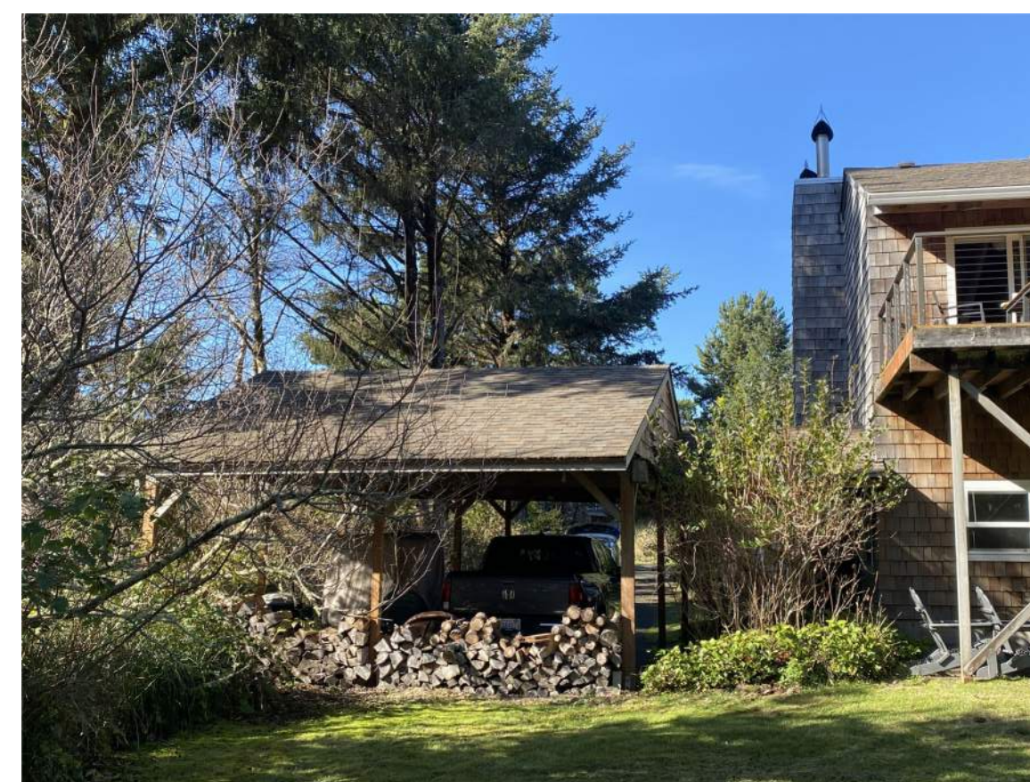
6 EXISTING CARPORT - REAR
