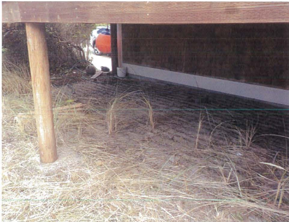
Photo 8 – Close-up view of the existing deck.
