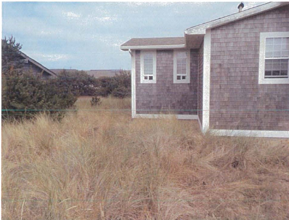
Photo 2 – Northerly view of the western side of the existing house towards the location of the proposed deck.
