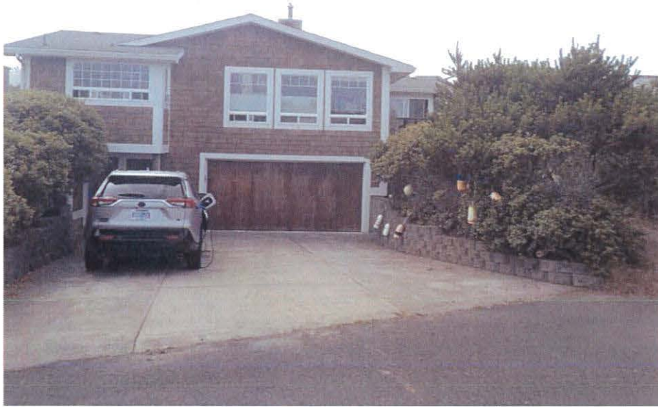
Photo 1 – Southerly view of the existing house at the site.
