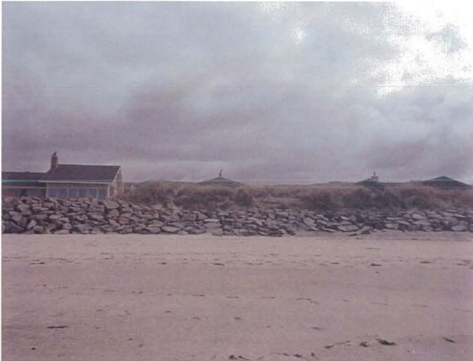
Photo 6 – Easterly view of the existing rip rap revetment exposed west of the site.
