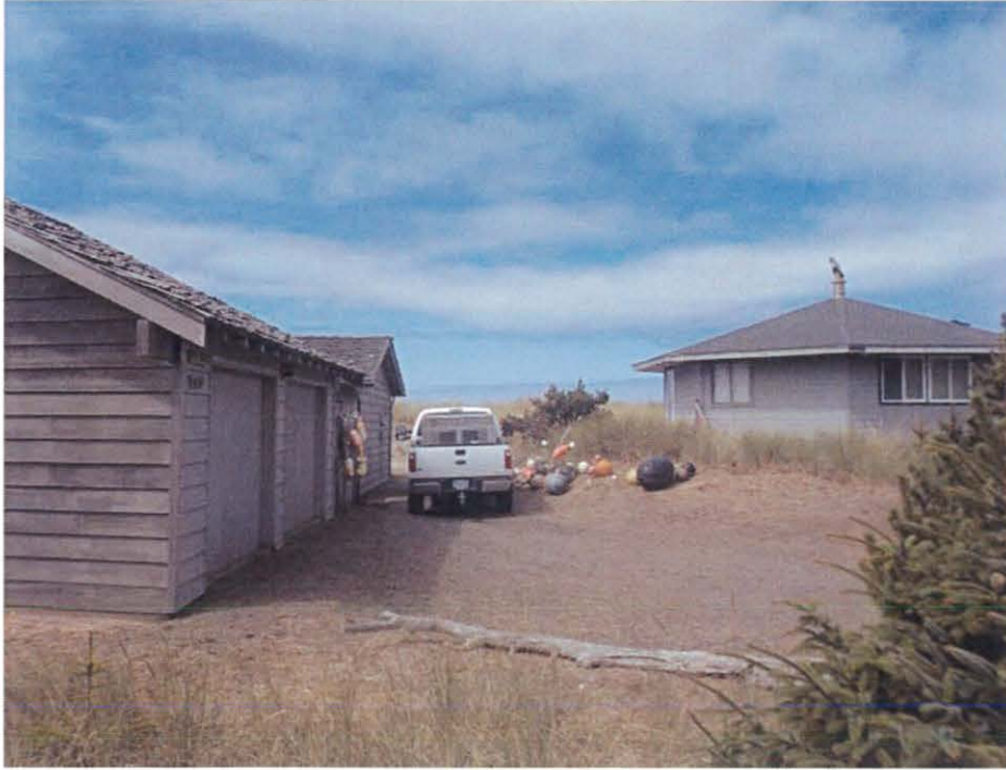
Photo 5 – Westerly view from the location of the proposed deck.
