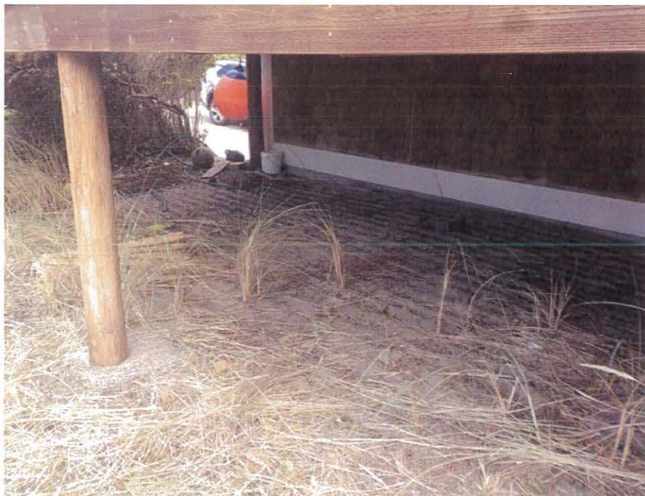
Photo 8 – Close-up view of the existing deck.
