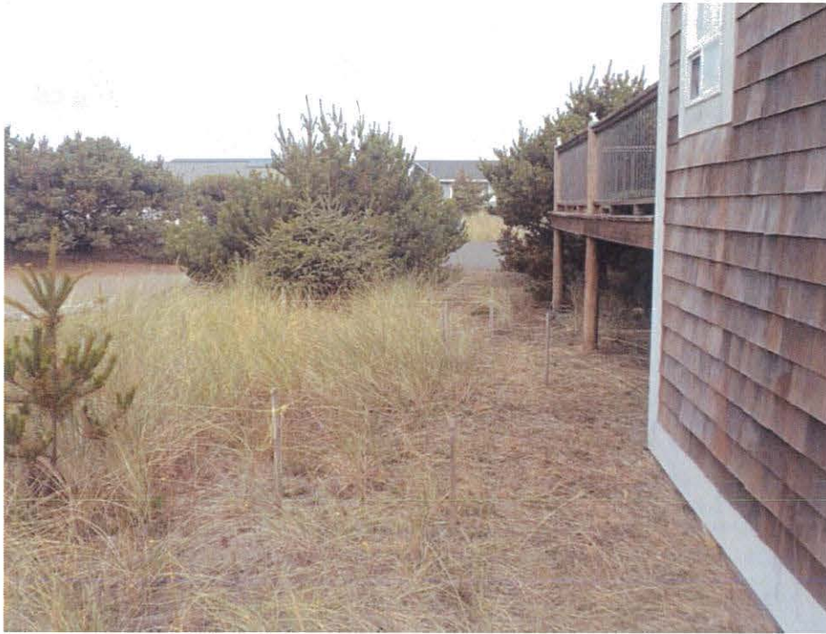
Photo 3 – View of the existing deck at the northwest corner of the house and the location of the proposed new elevated deck.
