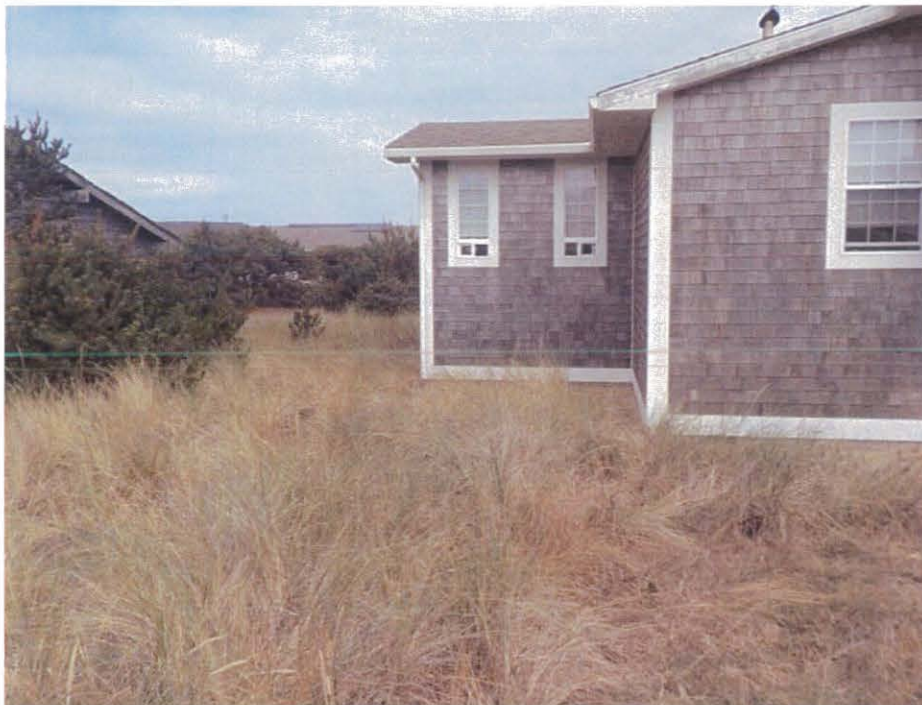
Photo 2 – Northerly view of the western side of the existing house towards the location of the proposed deck.
