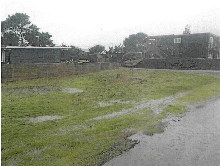
Photo 2 – Southwesterly view of the site from Amity Avenue.
