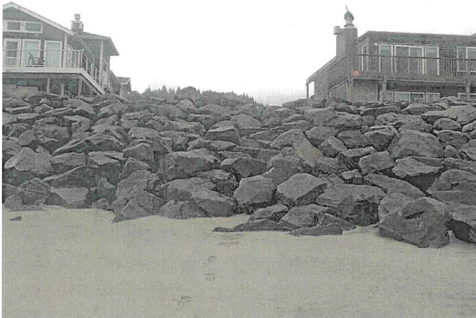
Photo 5 – Easterly view of the riprap revetment at the end of Amity Avenue near the site.
