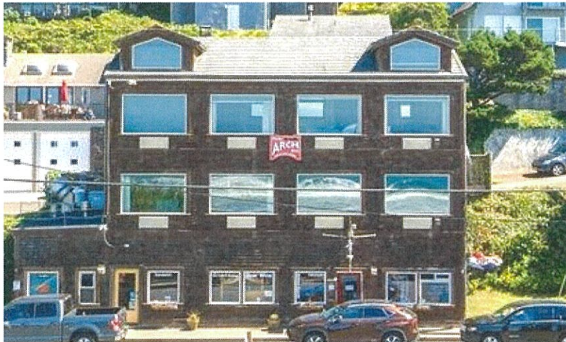
West Elevation of Three Arch Inn
