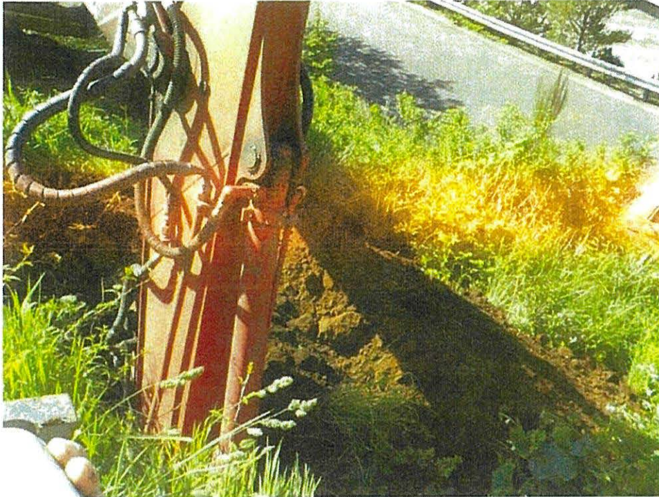
Photo 7 – View of Test Pit 2 being excavated (2018).
