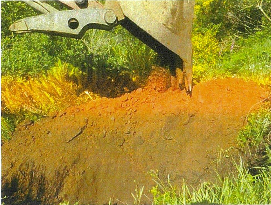
Photo 9 – View of spoils from Test Pit 3 (2018).
