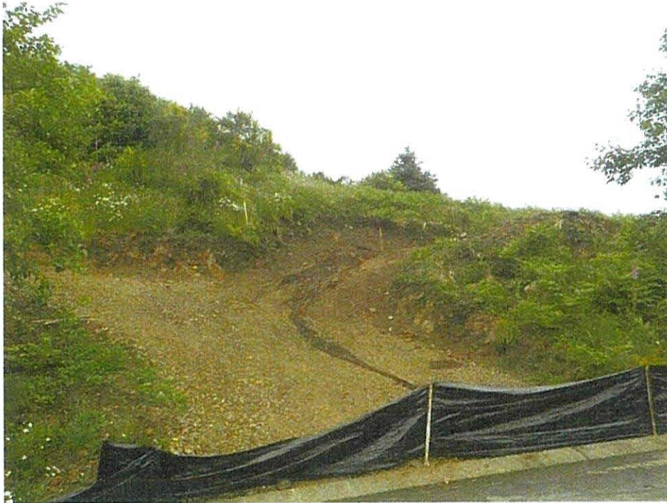
Photo 10 – Northeasterly view of the location of Boring B-1 from Tye Court (2019).
