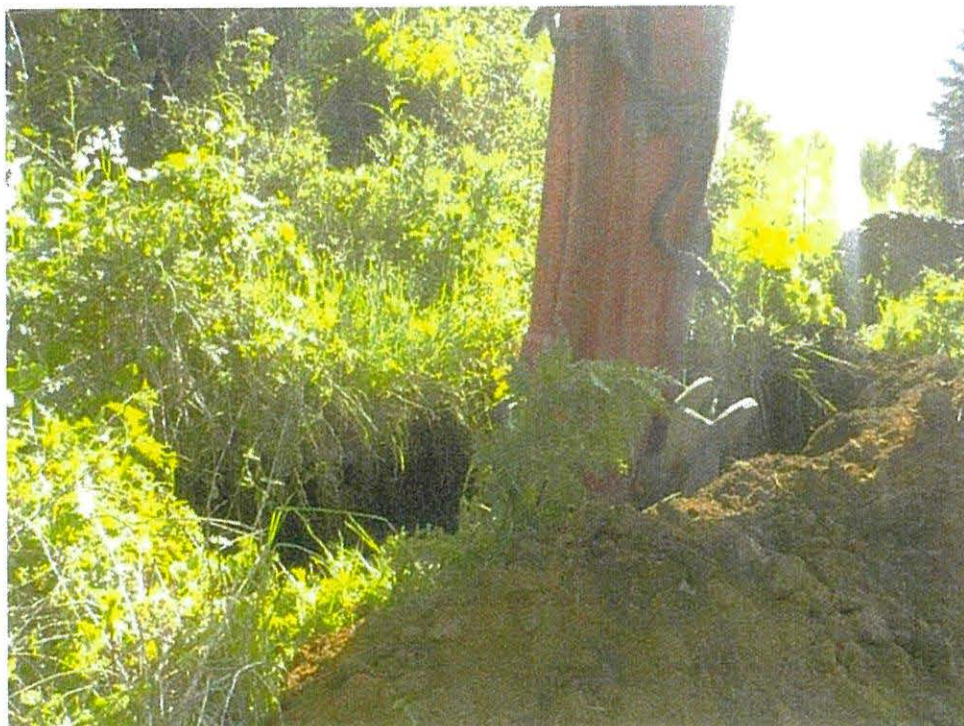
Photo 6 – View of Test Pit 1 being excavated (2018).
