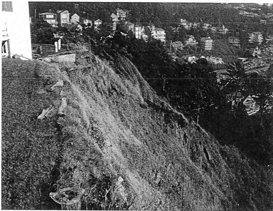
Photo 2 - Southeasterly view along the southern bluff slope.
