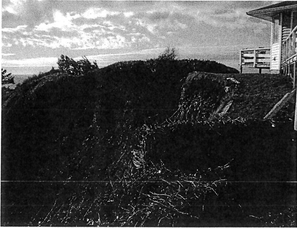
Photo 4 - Northwesterly view along the southern bluff. Southwest corner of existing building is at far lower right of photo.
