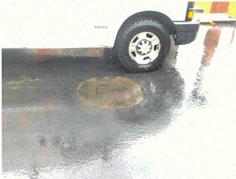
Photo 8 – Close-up view of a manhole near the site indicating the potential presence of buried private utilities and installations.
