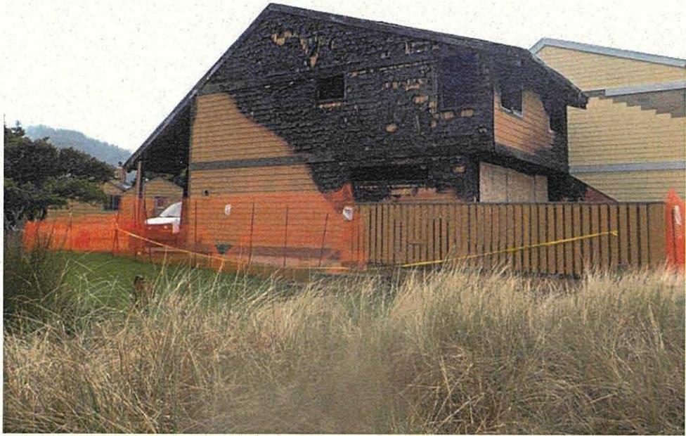
Photo 3 – Southwesterly view of the subject site from near the intersection of Breakers Blvd and Mt. Angel Ave.
