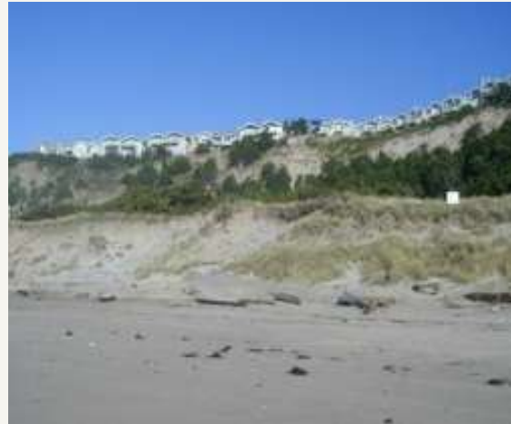
Figure 31. Erosion at “The Capes” Condominiums, Oceanside, Oregon
