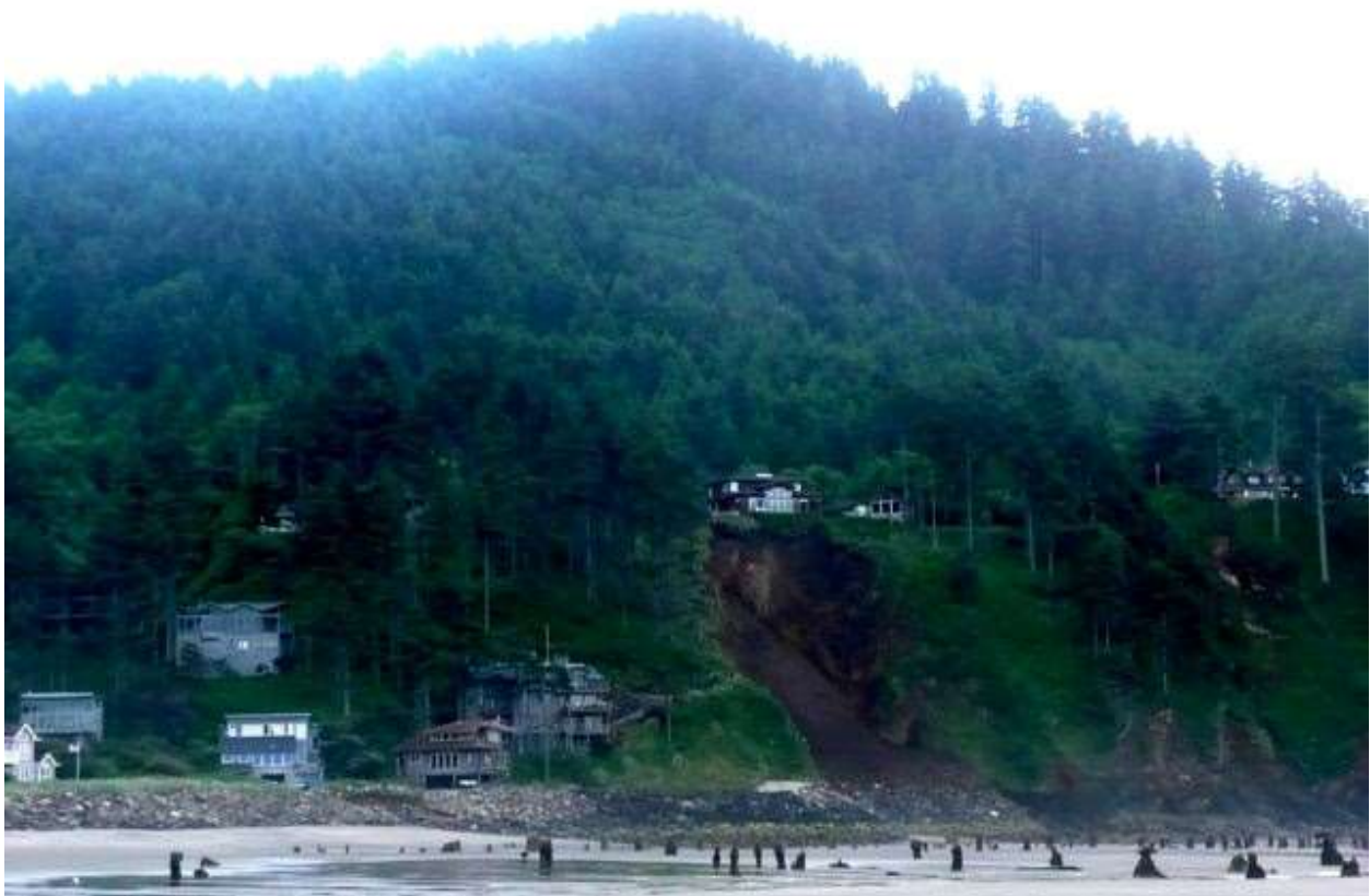
Figure 63. Landslide in Tillamook County
