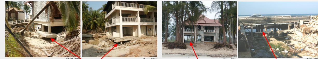
Foundations undermined by scouring
