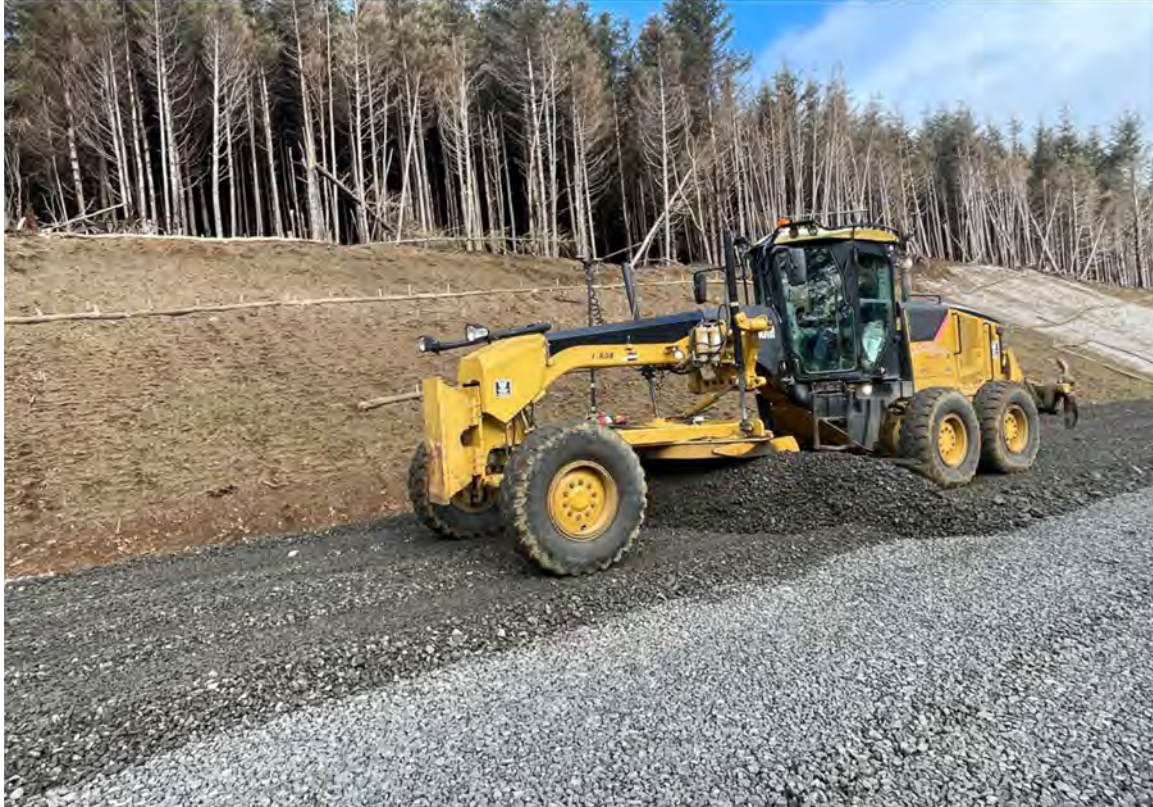
View of grading newly placed roadway aggregate.
