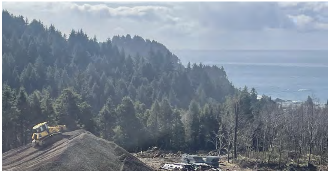
View of stockpile near South project entrance.
