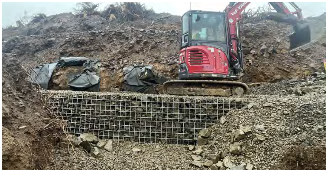
View of MSE Wall No. 2 after the placement of two courses.
