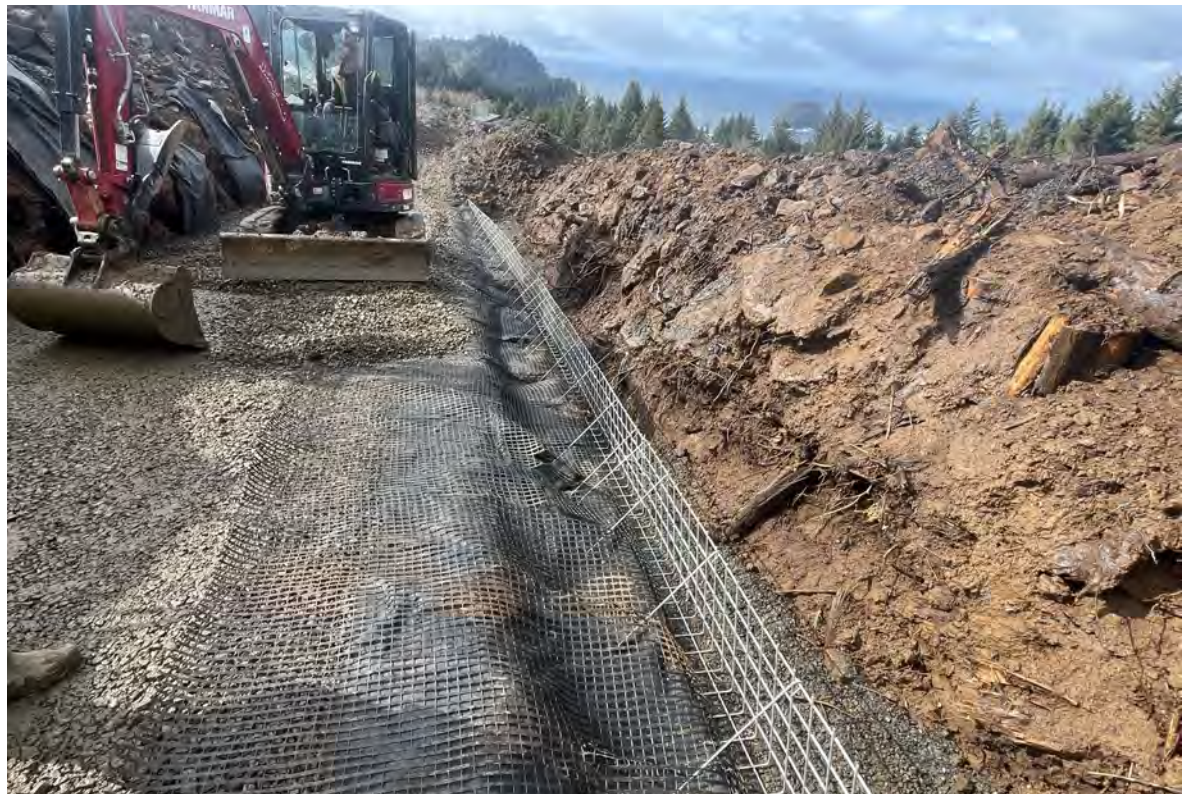
View of the first course of MSE Wall No. 2 near completion.
