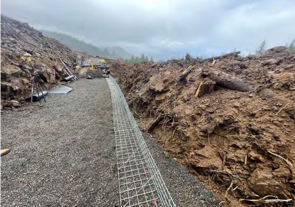
View of first course preparation of MSE Wall No. 2.
