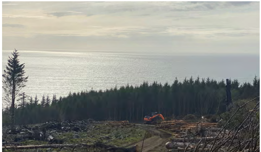
Processing timber at station 365.
