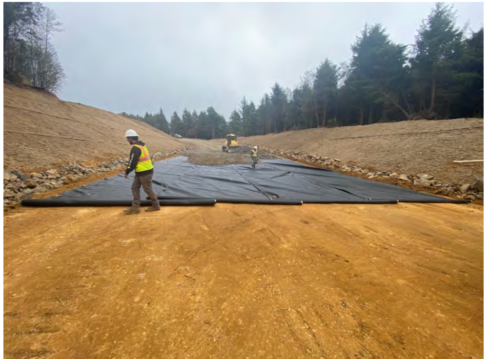
Placing select borrow over subgrade
