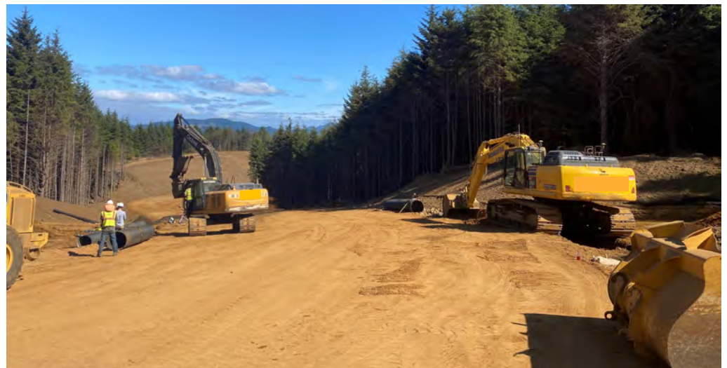
Installing culverts
