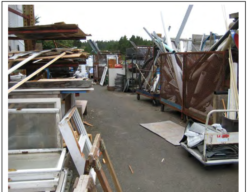
Building material reuse area at Manzanita Transfer Station, photo taken September 12, 2011.
